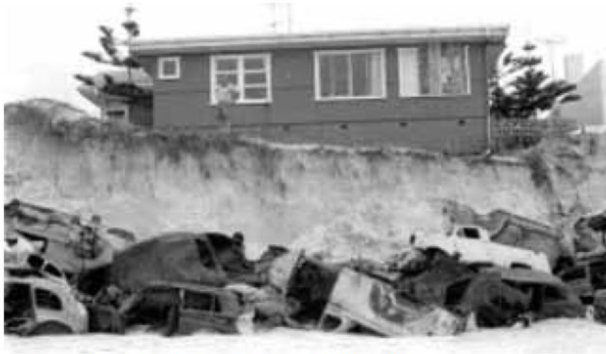
Car bodies used to try and stop the progress of erosion on the Gold Coast, 1967.
